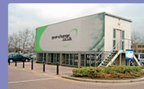
Shower block and cycle parking combined
