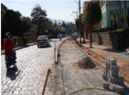
The cycle way under construction
