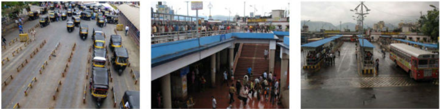
Figure 70. Thane Suburban station in India with lower level for auto-rickshaws and upper levels for bus bays. It connects to the road level via elevated walkways (Source: WRI India)
