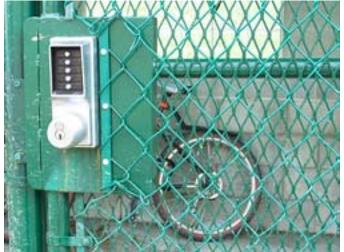
An electronic key pad is one option for a bicycle cage. Periodically resetting an access code will further improve security. Photo credit: John Luton.
