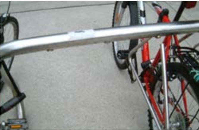
Choosing inappropriate materials will compromise security. Welded sections of this stainless steel rack have been broken off by vandals or thieves.
