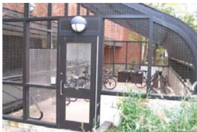
Bicycle cage at Toronto Reference Library (Glass roof extends down from main building, wire mesh walls, restricted access through electronic key pad).
