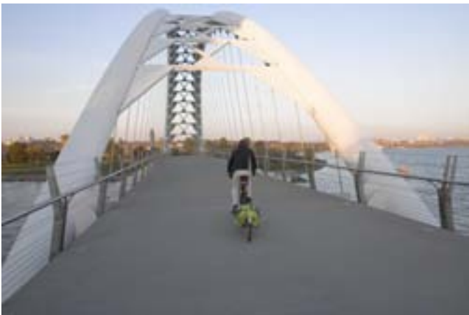
Humber river pedestrian and bicycle bridge
