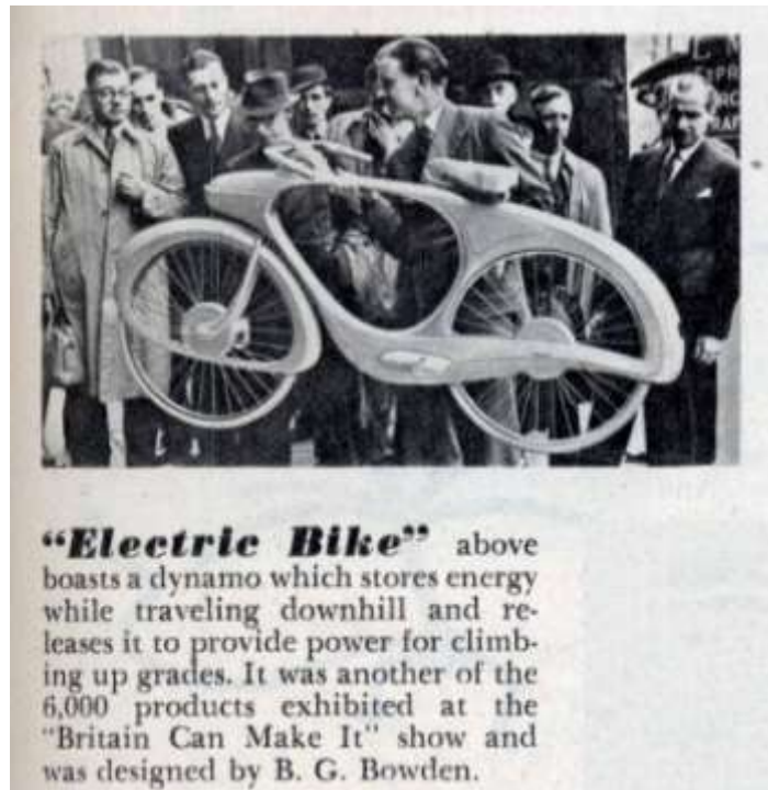
Figure 9: 1947 Bowden Fibreglas electric Bicycle
