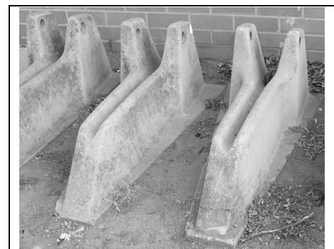
Figure 3 – An Example of Unacceptable Parking Installations
